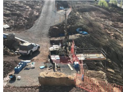
B1.1 Borehole drilling (P193 - cantilever)
