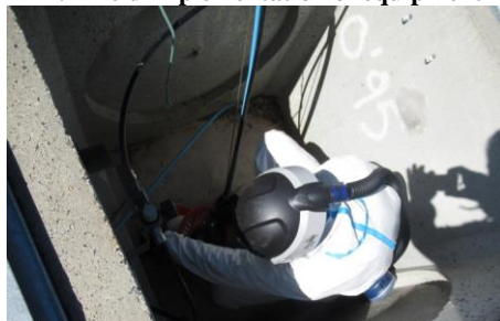
B1.3 Field works during the tracer tests
