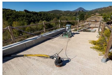
B2.1 Barrier boreholes for aeration
