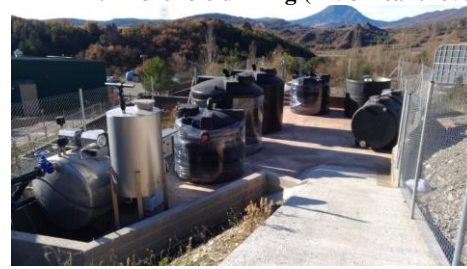
B1.2 Field implementation of equipment
