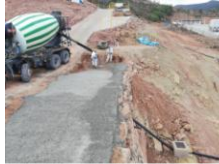
B1.1 Construction of borehole platforms
