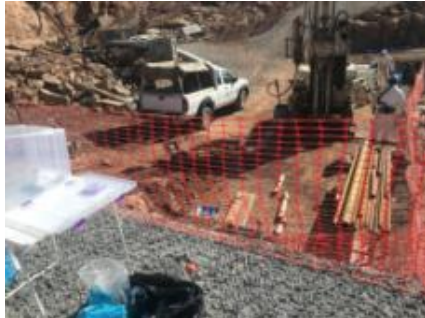
B1.1 Borehole drilling
