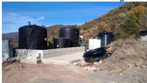
B1.2 Field implementation of equipment
